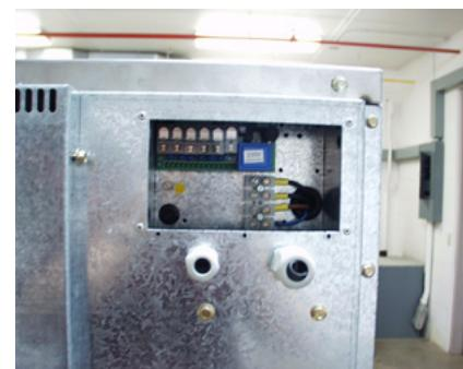
8. Verify that the insulation is intact on all external wires and that all connections are secure. If bare wire is evident, call a service technician.
